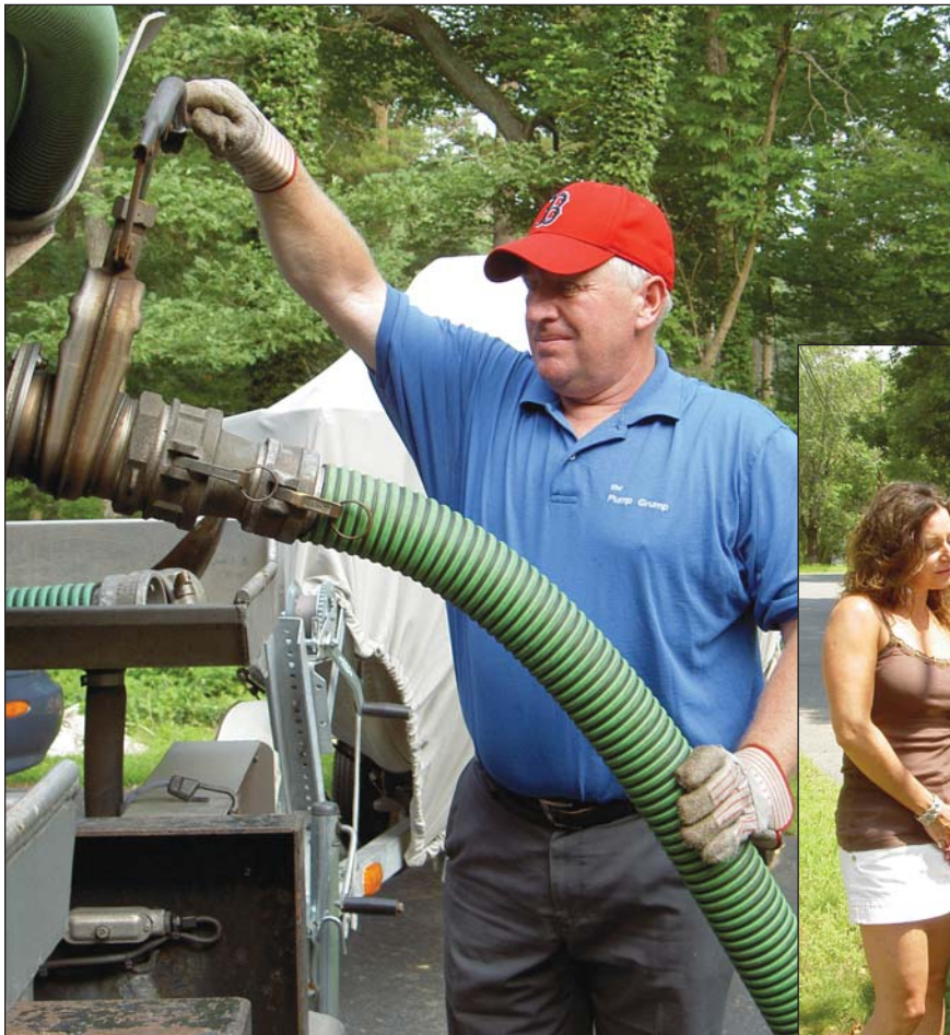
Above, Buddy Juergens closes the tank valve after pumping a septic tank. Right, Juergens explains septic cleaning charges to a customer. Before he leaves a jobsite, Juergens makes sure customers understand all work performed and maintenance recommendations.
